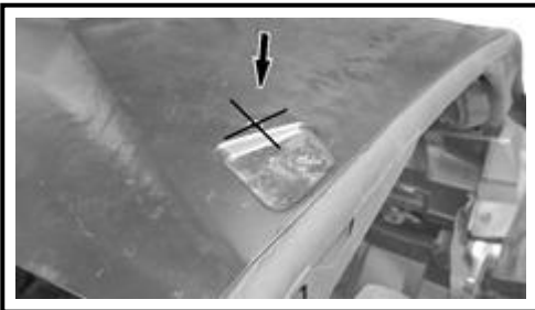
TYPICAL - FRONT LEFT CORNER OF ROOF
